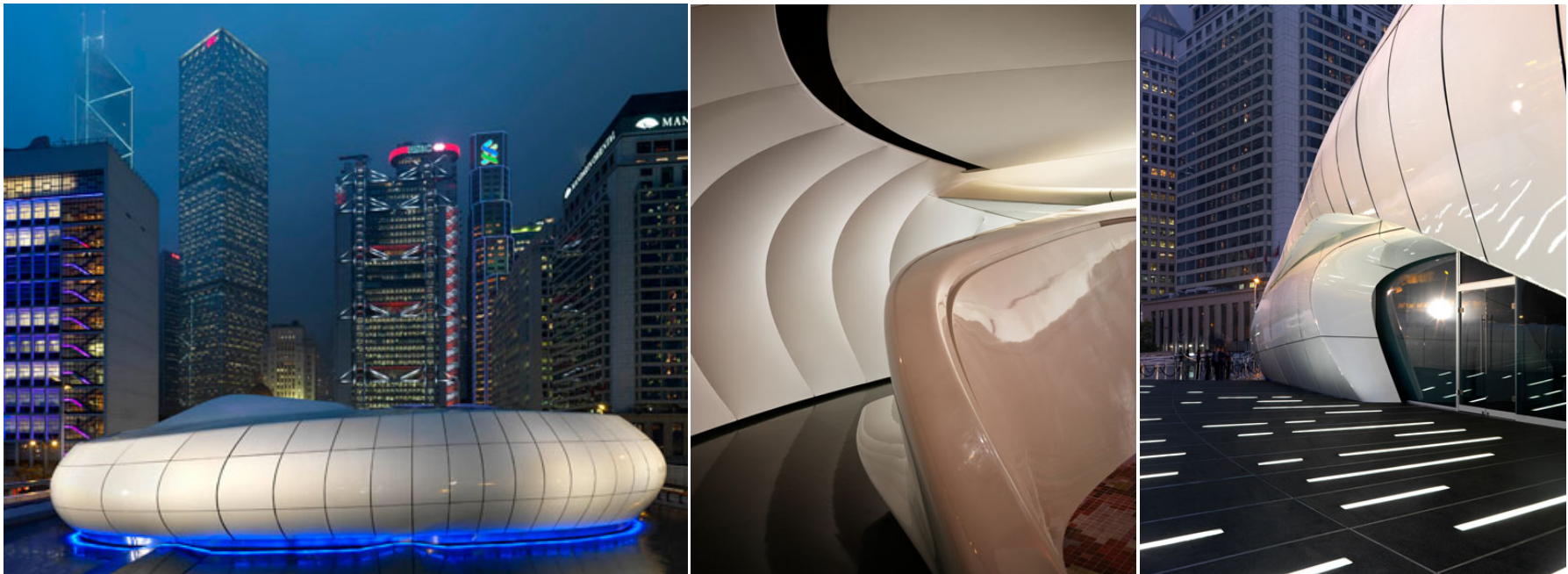
Hadid's Chanel pavilion made entirely from Plug&Play components and assembled and disassembled in Tokyo, Hong Kong, New York
